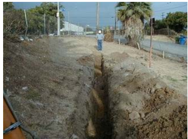
Trench Dug for Soil Sampling
