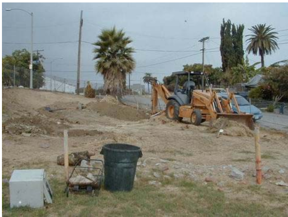
Backhoe Digging Trench for Site Investigation
